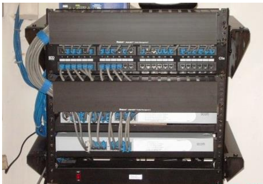
Figura 30: Rack de pared
