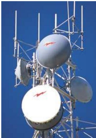
**Figura 0.6 Antenas microonda**
